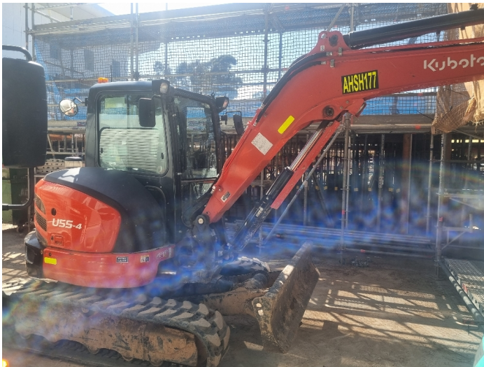
Overall View - Right hand side
